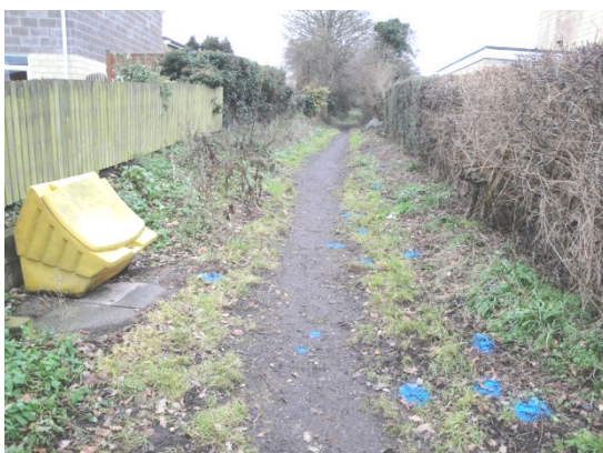
Byway 89 Before Surfacing
